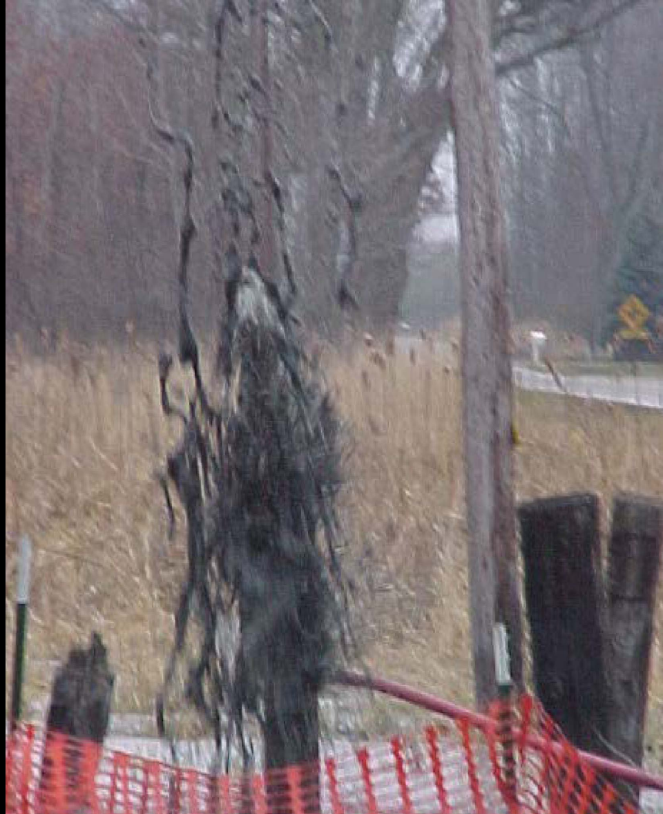
BLOWING OBSTRUCTING SOIL & DEBRIS OUT OF THE WELL
