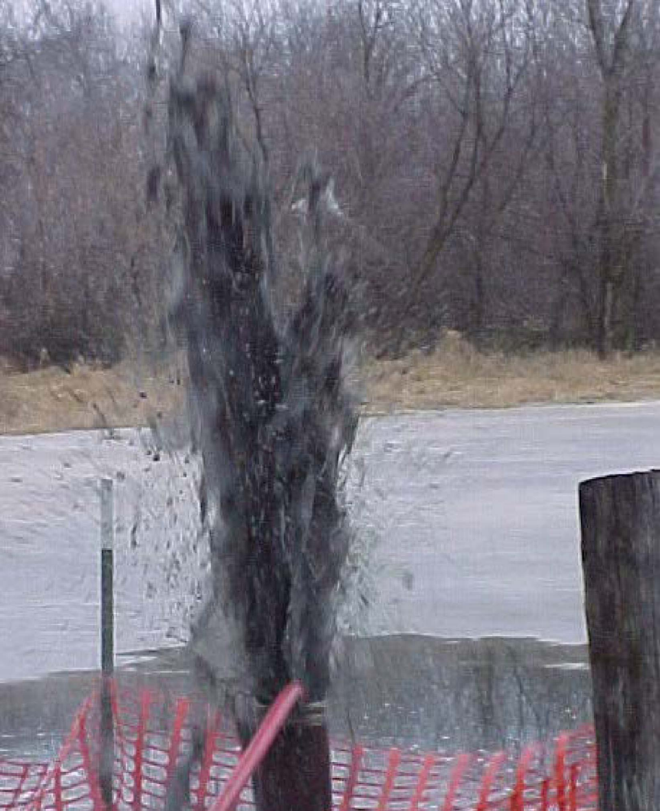
BLOWING OBSTRUCTING SOIL & DEBRIS OUT OF THE WELL
