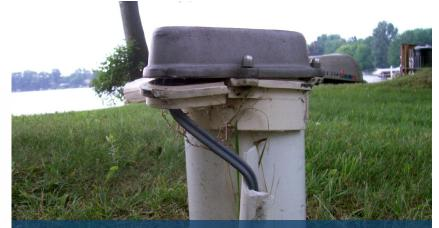
Damaged wellhead with cracked well cap and exposed wires Photo provided by Barry-Eaton District Health Department
