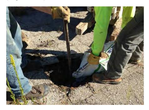
Finally, the surface at each location was restored to a similar condition. In the gravel covered areas, the final six inches were filled with gravel. In the asphalt area at OW-9, the final six inches were filled with concrete (see photo below).
