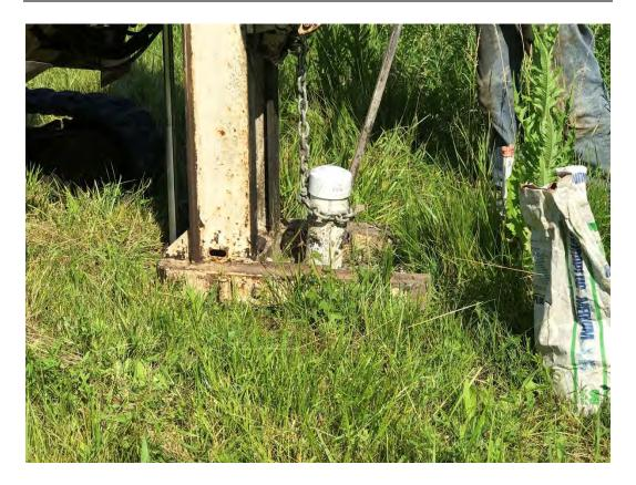
Next, the one-inch diameter PVC well screens and casings were removed from the ground with the assistance of the Geoprobe track rig (a chain was placed around the well and the hydraulic hammer from the track rig was used to pull the well out of the ground, see photo above). Tubing associated with the soil vapor probe was detached from the vapor probe and pulled from the ground.
