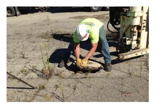
Next, the two-inch diameter PVC well screens and casings were removed from the ground with the assistance of the Geoprobe track rig (a chain was
