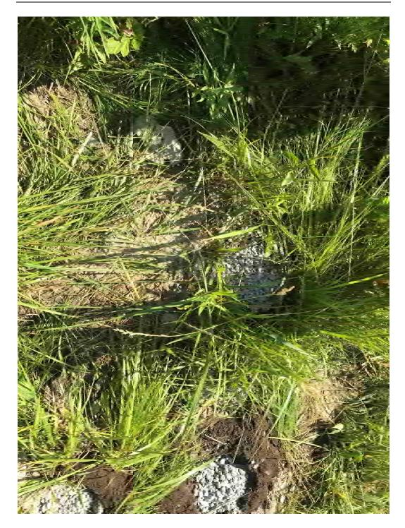
Finally, the surface at each location was restored to a similar condition. Fill sand was placed over the around the former borehole (see photo below).
