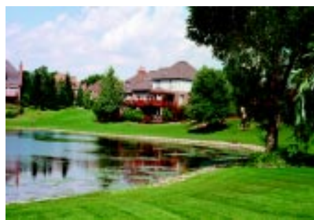
Wet Detention Basin
