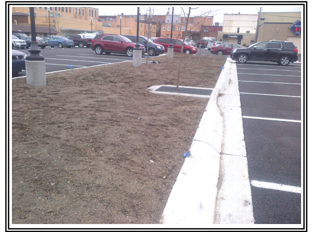
Site After: Vegetated Swale with Tree Box Filter in Finished Parking Lot
