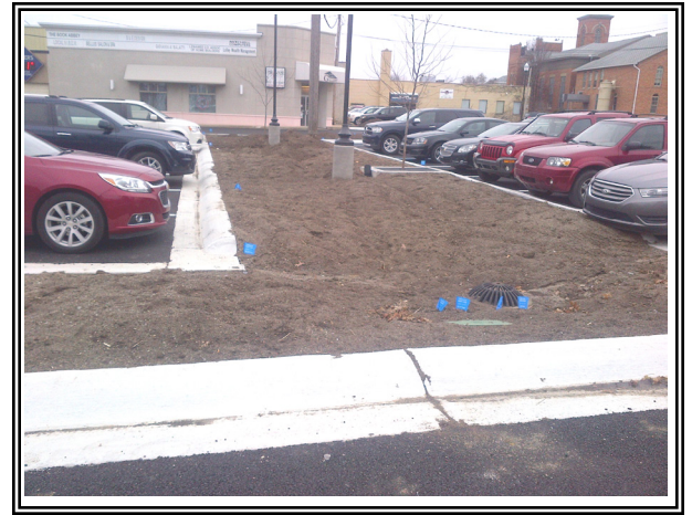
Site After: Vegetated Swale in Finished Parking Lot
