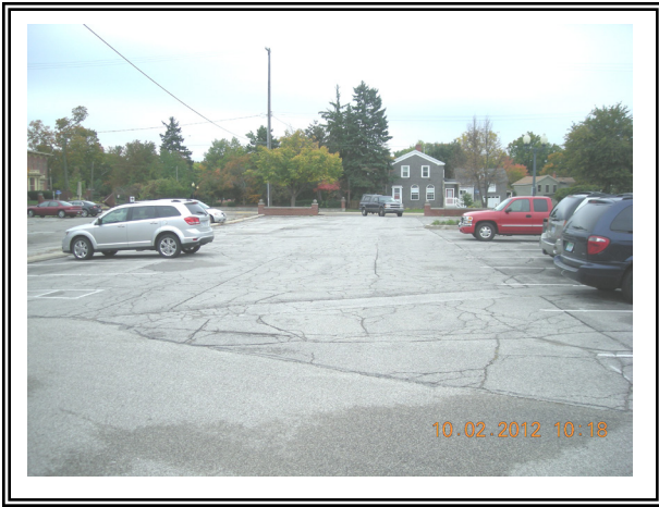
Site Before: Parking Lot
