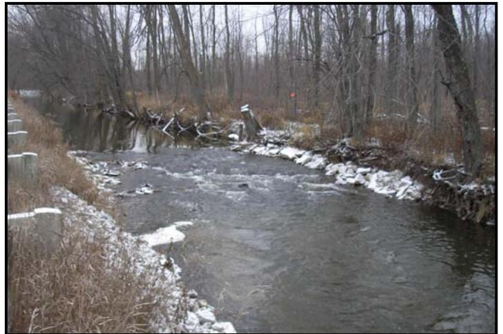
**After:** Riffle structures were installed to improve water quality by reducing bed and bank erosion, centralizing the flow away from the banks and increasing aquatic habitat diversity.
