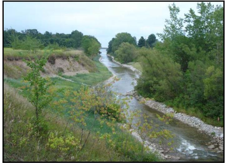
**After:** A new channel was created through a process of cutting and filling within this portion of the project area. Rock riprap in the form of Newbury Riffles and bank armoring was keyed into the drain bottom and placed up the side of the channel to a height equal to the bank-full elevation. A floodplain shelf was constructed from the top of the new channel banks outward to the sides of the existing valley walls.
