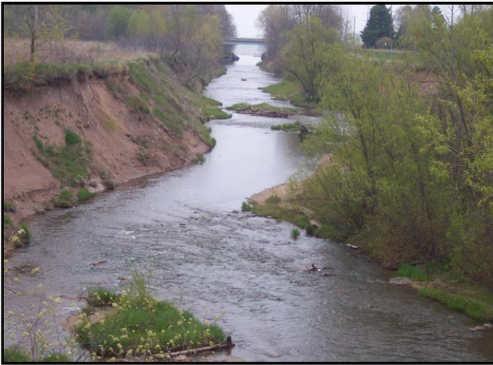
**Before:** Originally a 3' x 2' channel, excessive erosion, down-cutting, loss of floodplain and in-stream deposition created the 110' x 40' channel (pictured above). The impaired watercourse contributed the highest sediment bedload of any watershed in the Saginaw Bay region. Due to the excess bank erosion and associated sedimentation, water quality and aquatic habitat was severely degraded, and migration for the many species of fish that use this river for spawning was compromised.
