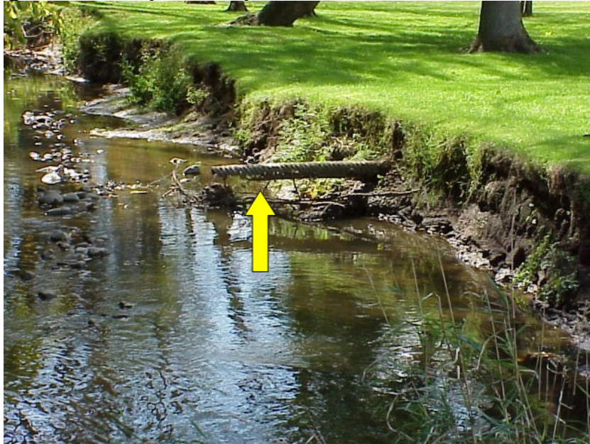
Figure 6. Example of Exposed Infrastructure in a Channel.
