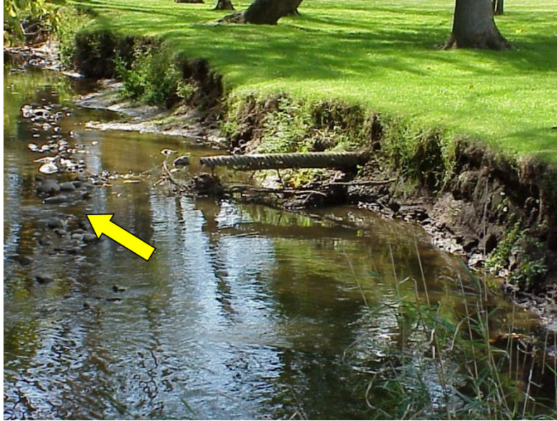
Figure 10. Example of Failed Bank Stabilization BMPs.
