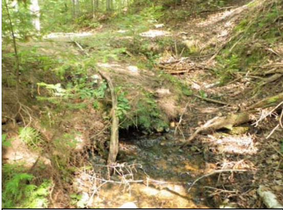
Figure 6. Groundwater seep downstream of Silver Lake Road at the Little Ocqueoc River.
