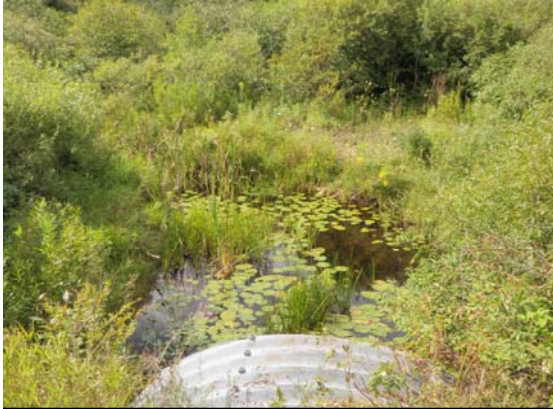
Figure 20. Tomahawk Creek downstream of County Road 634.
