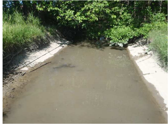
Figure 7. Concrete-lined Smith Creek at Gibraltar Road.
