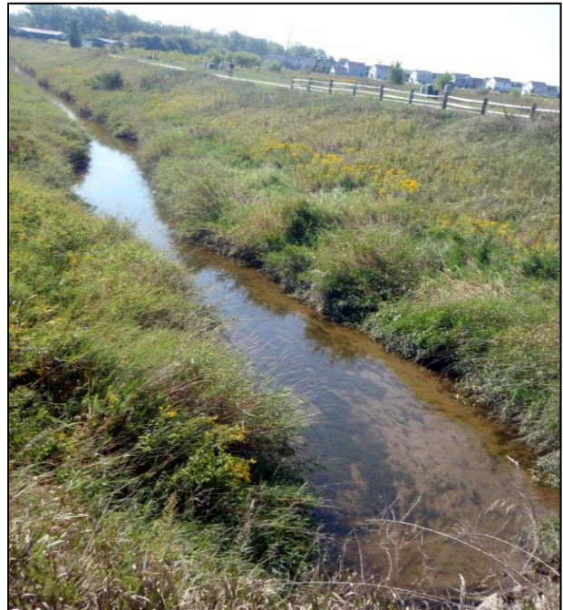
Figure C: Remy-Chandler Drain upstream of State Road.
