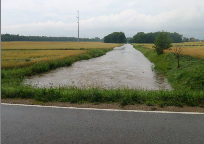
Photo E: High water conditions downstream Bad Axe Creek July 2013.
