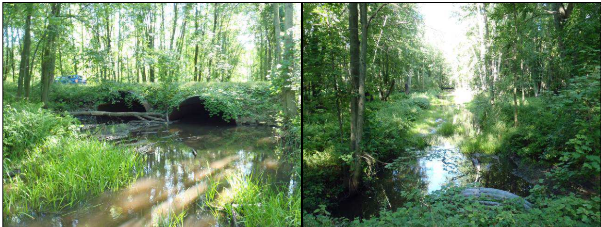
Alder Creek Drain at Tisdell Avenue.
