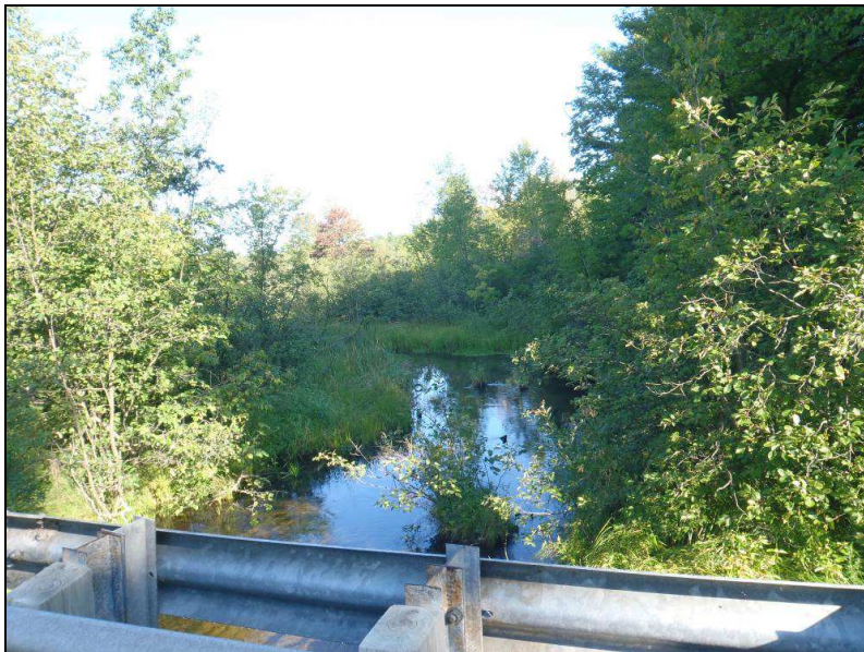
West Branch Creek at Stanton Road.
