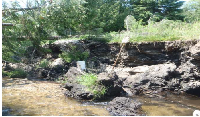
Figure 3. Significantly eroding banks were observed in 2013 upstream of Springbrook Road on the north branch of the Boyne River.
