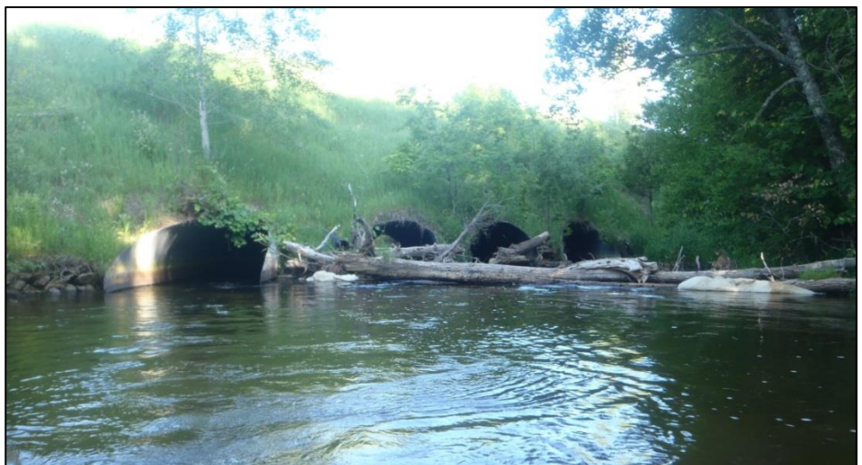
Figure 15. Station 9, Betsie River upstream of Kurick Road looking downstream with a four-culvert road crossing.
