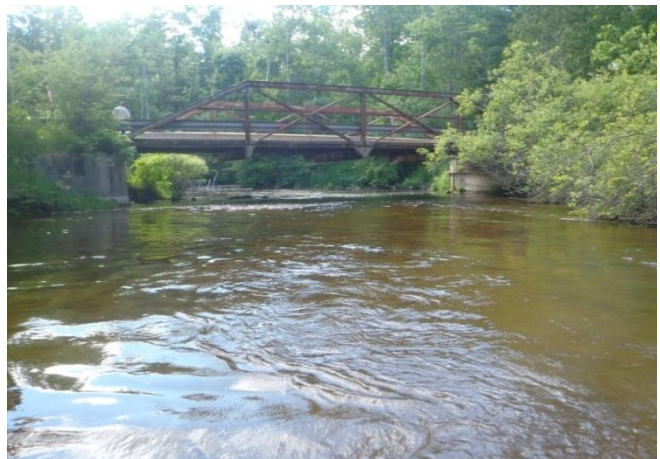
Figure 7. Station 8, Betsie River upstream of Haze Road looking downstream at an old iron bridge crossing.
