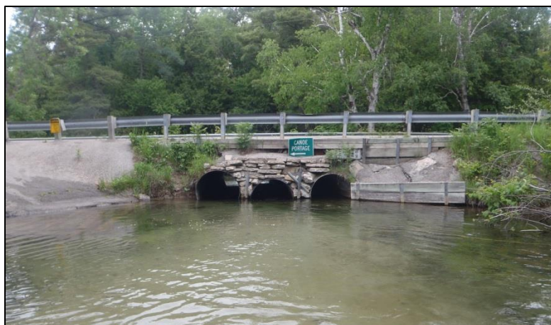
Figure 13. Station 1, Crystal River upstream of Crystal View Road looking downstream at crossing.
