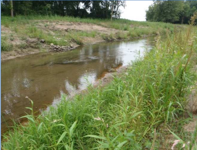
Figure 2. Station 13, Black Creek Downstream of 144th Avenue. Heavy sand deposition.
