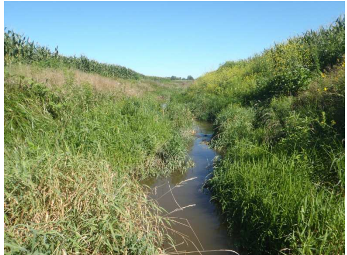
Figure 9. South Branch Macon Creek at Pocklington Road.
