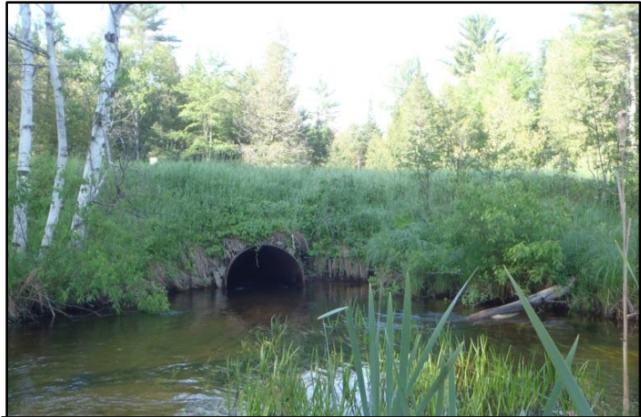
Figure 7. Upstream of Fife Lake outlet looking at East County Line Road crossing
