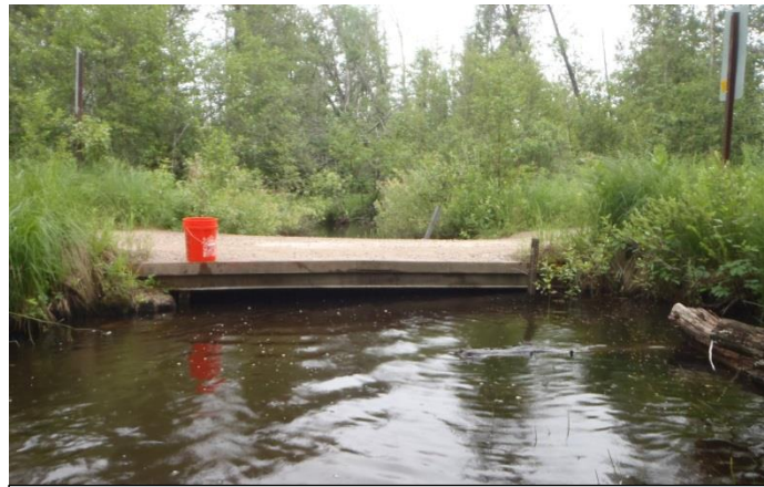
Figure 8. Road crossing over Anderson Creek at County Line Road.
