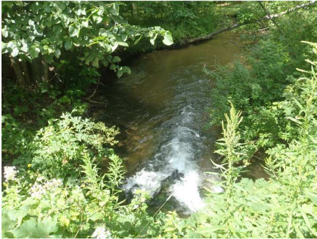
Figure 9. Perched culvert in Sanborn Creek, looking downstream at Spruce Road (Site 13T).
