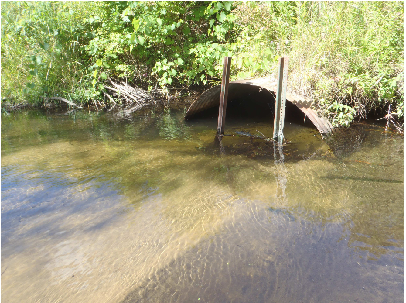
Figure 8. Water and sediment tend to accumulate upstream of under-sized culverts, as seen here on Sanborn upstream of Foreman Road (Site 15).
