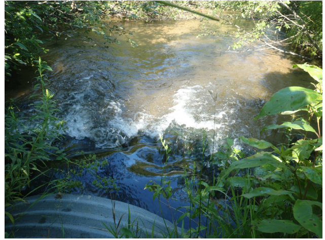
Figure 10. Perched culvert in Sanborn Creek, looking downstream at Broadway Street (Site 14T)
