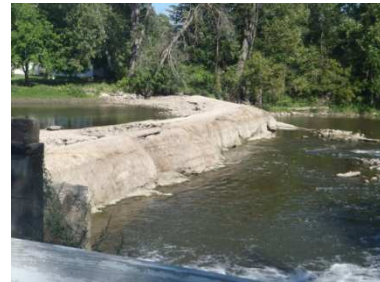
Corunna Dam, September 2015
