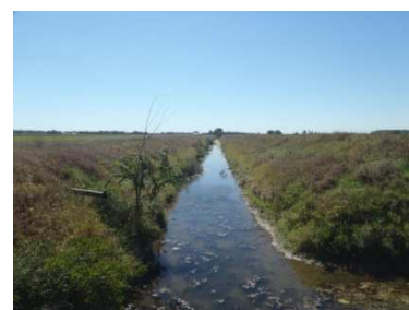
Carson Drain (Ryan Road) 2015
