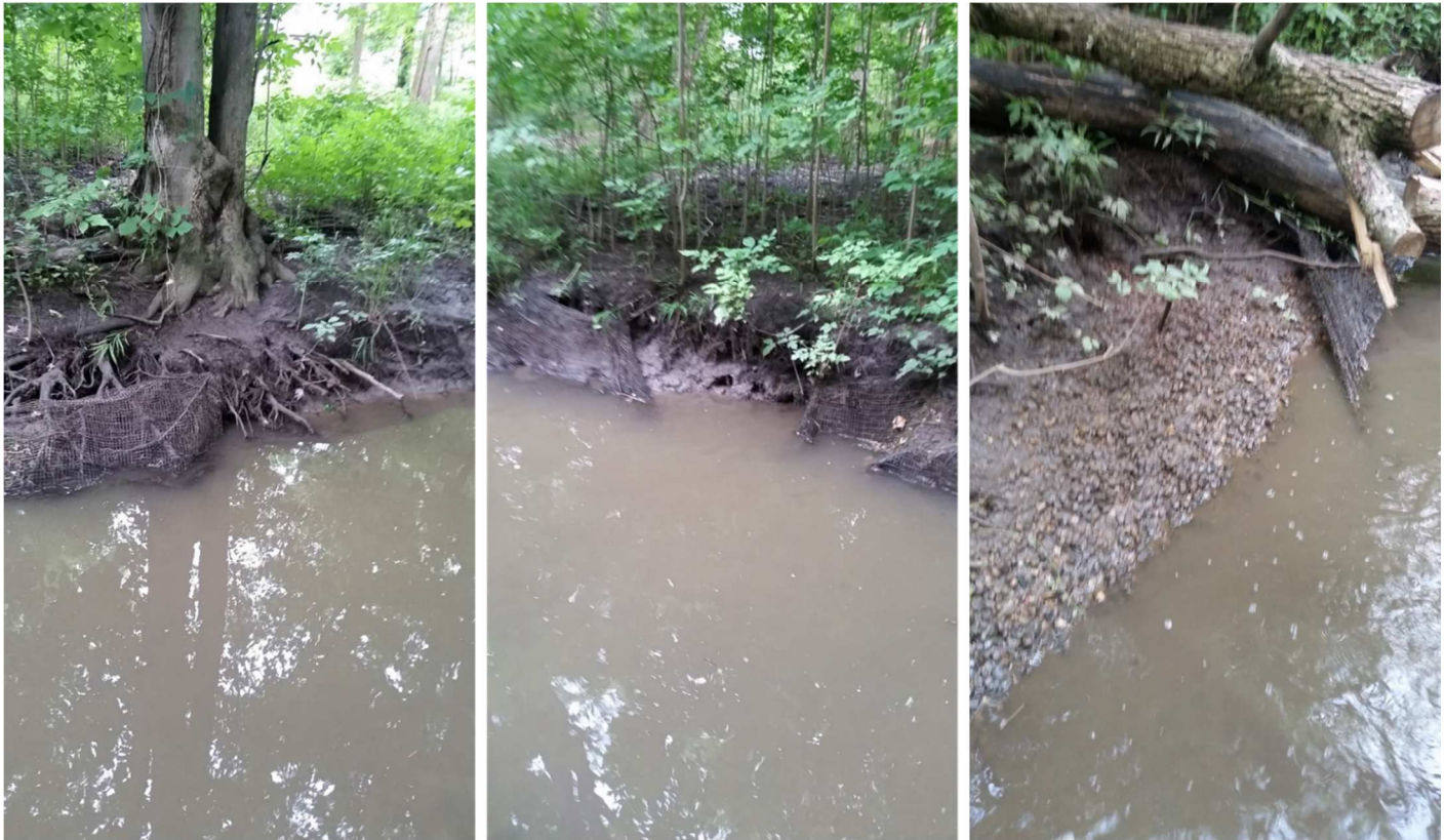
Figure 6. Exposed erosion control netting along banks at Station 1.
