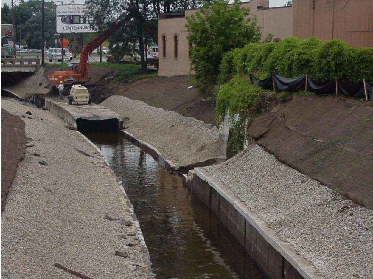
Figure 2. Concrete cap being removed from over top of the Grand River in downtown Jackson in 2000 (photo by K. Price, https://rodmalloy.com/tag/kenny-price/ ).
