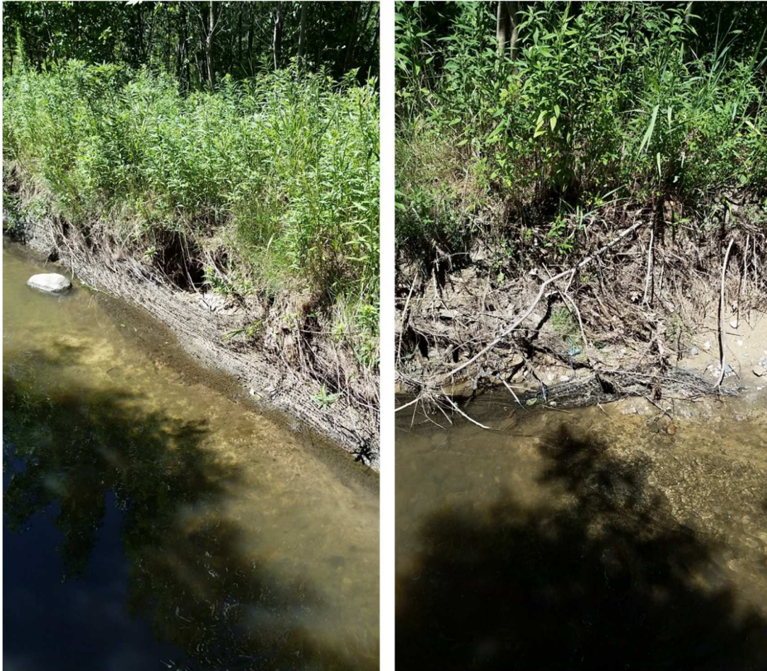
Figure 7. Exposed erosion control netting at Station 11.
