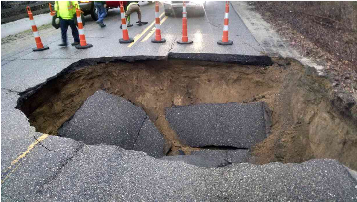
Figure 2. Collapsed section of 148th Avenue in Spring Lake Township after a culvert failure. Image from: (The link provided was broken and has been removed.)
