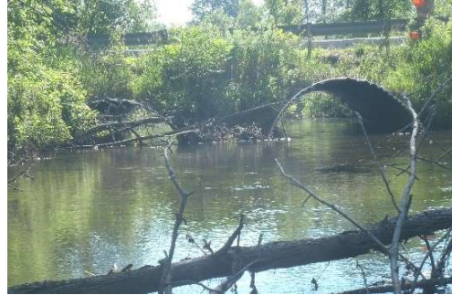
Figure 23. Culverts for Fish Creek crossing at Vickeryville Road, Clinton County, Michigan, July 2017.
