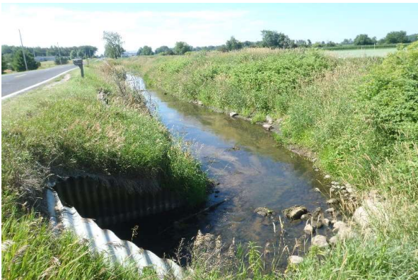
Figure 2. Little Maple River upstream of St. Clair Road, Clinton County, Michigan, July 2017.
