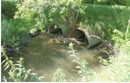
Figure 22. Undersized culverts for Fish Creek at Pine Grove Road, Clinton County, Michigan, July 2017.
