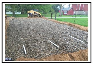
Garfield Street After: New septic tanks and a raised mound pressurized drain field were installed, allowing all waste water to be properly stored and treated.
