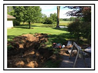
Warner Street Before: The drain field on this site was in failing condition. It was not properly treating effluent, causing untreated waste water to drain into the nearby creek.
