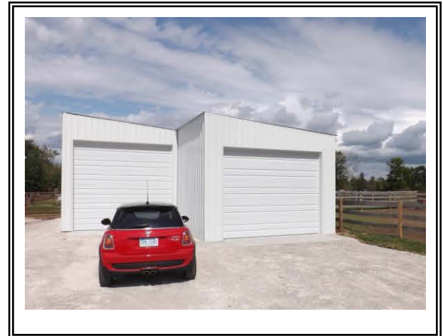
Manure Shed After: Extension to manure shed allows all manure to be covered and a concrete pad to store it on and scoop to transfer.
