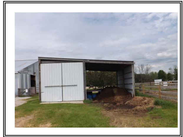
Manure Shed Before: Pile of horse manure was exposed to rain and snow, allowing nutrients to flow into the nearby ditch.
