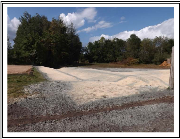
Horse Crossing Construction: Area was cleared to install exclusion fencing and the crossing stabilized with mulch blankets. Construction took place during dry weather when no water was present in stream.
