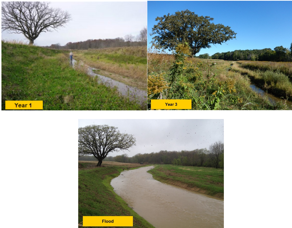
Figure 3. Bradley Drain one year and three years post-construction of a two-stage ditch during base flow conditions (top) and during high flow after rain (bottom).
