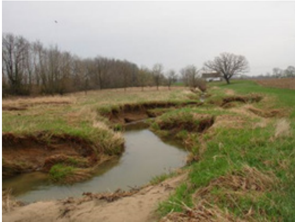
Figure 1. Before construction picture of Bradley Drain with extensive stream bank erosion.
