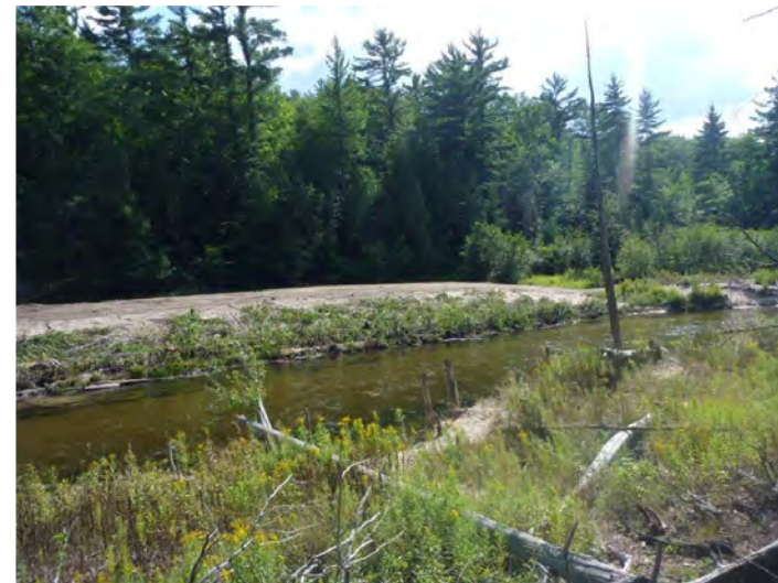
Figure 2. Technique 2. In many places, vegetation was established along the bank toe, so the bench was simply excavated behind the vegetation. This photo shows the toe vegetation being preserved and the transplants being placed on the excavated bench.
