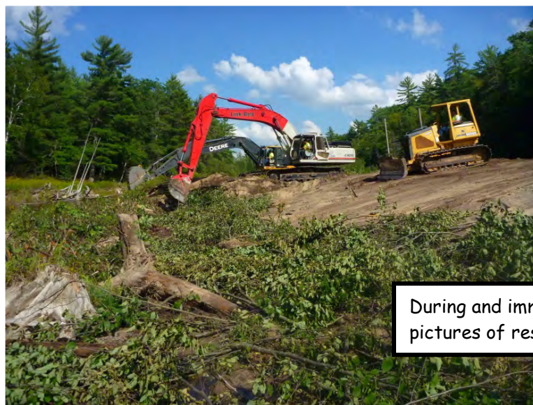
Figure 2. Technique 2. In many places, vegetation was established along the bank toe, so the bench was simply excavated behind the vegetation. This photo shows the toe vegetation being preserved and the transplants being placed on the excavated bench.
