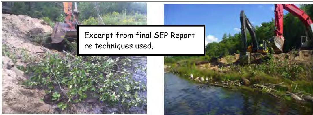
Figure 1. Technique 1. Bank is excavated and the tops of alders are placed underneath transplants. Technique 1 is used when the toe is devoid of vegetation.
