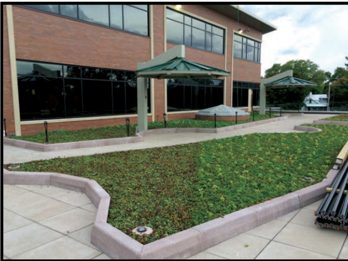
MMC's Cowell Family Cancer Center - green roof and infiltration trenches
