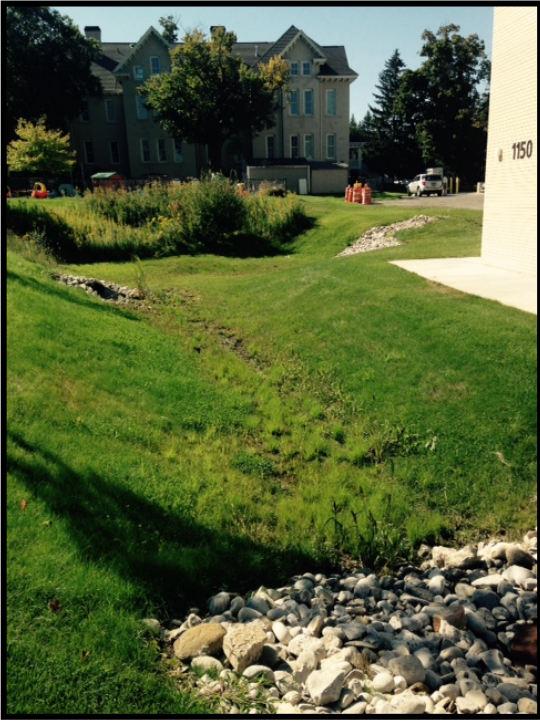
MMC's Building 29 - rain garden retrofit
