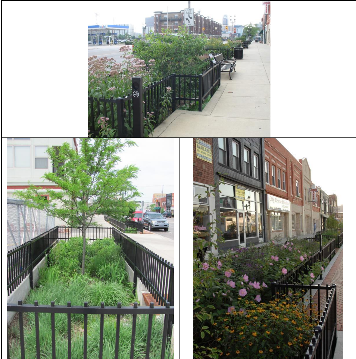
Figure 1. Photographs of the rain gardens.
