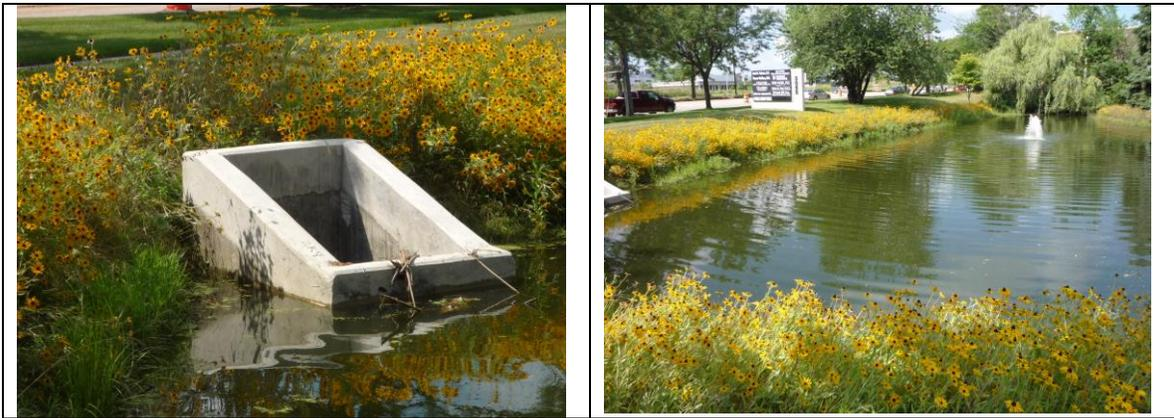
Figure 3. Retrofitted storm water detention pond, 1 year after installation.
