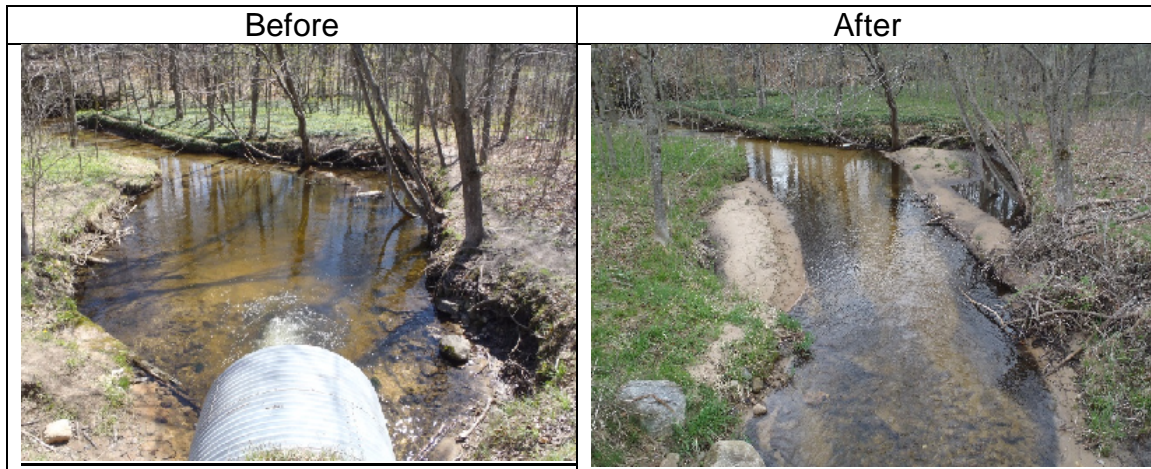
Figure 2. Before and after photographs of Osborn Creek downstream of the Pierce Road culvert, showing the plunge pool and destabilized stream channel (before) and the narrower, shallower channel and floodplain benches (after).
