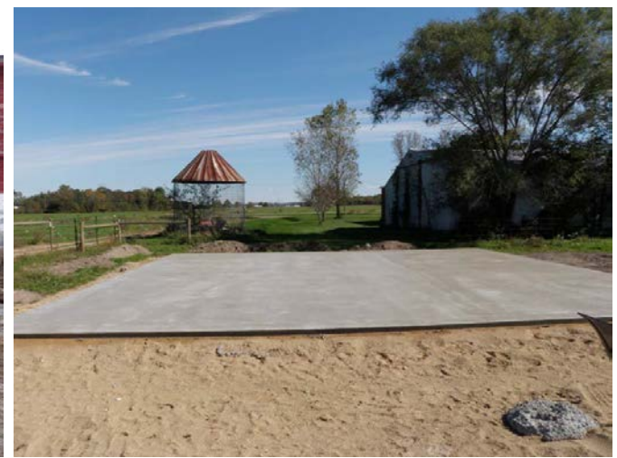
Farm on Pierce Drain: After Photos of well trough and heavy use protection installed to reduce animal access erosion.
