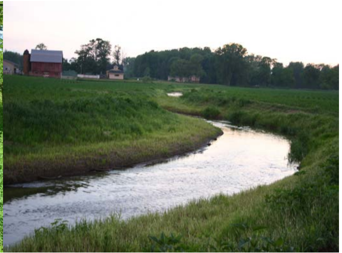
Murphy Drain After: Multi-Stage Channel installed to create bank stabilization & reduce sediment flow.
