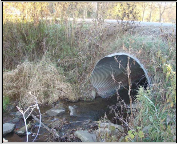
26 th Street Culvert Before: Poorly aligned and undersized culvert caused persistent erosion. The culvert was also subject to blockage causing damage upstream.
