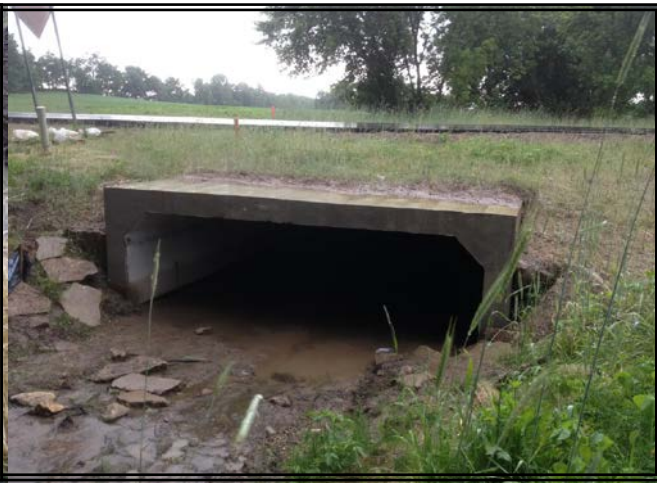
146 th Street Culvert After: Box culvert installed to lower erosive energy during high flow events. Bank reinforcement has stabilized the area.
