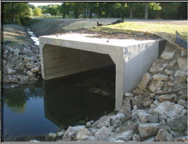
26 th Street Culvert After: Box culvert was installed to lower erosive energy, align with stream flow and allow unrestricted water passage. Critical areas of the stream banks were reinforced to prevent erosion.
