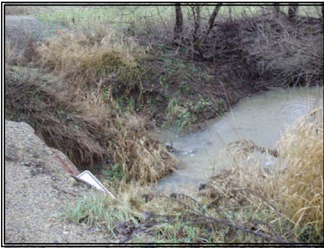
146 th Street Culvert Before: Unstable roadside bank with culvert barely extended beyond road's edge. Flashy stream with high flows after rain falls.
