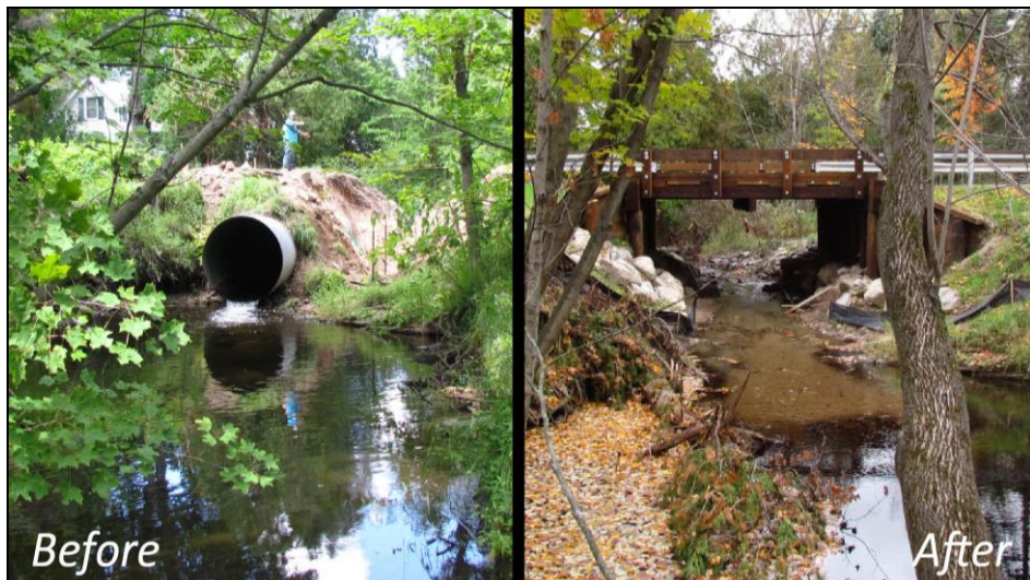
The before picture shows the perched culvert under Pierce Road at Cobmoosa Creek in Oceana County. The after photo shows the timber bridge spanning the creek, allowing free-flowing condition, and reducing flashiness and bank scouring. The surface of the bridge and the approaches on both sides were paved, further reducing sedimentation.
