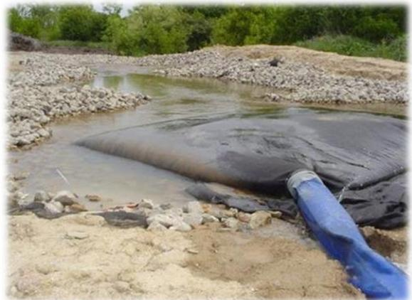
For very small sized sediment particles, such as fine silts and clay, polyacrylamides (PAMs) must be used in conjunction with other sedimentation controls such as filter berms, filter bags, sedimentation basins, geotubes, and geojute. PAMs bind with the sediment particles forming a flock that settles out of the water column.
