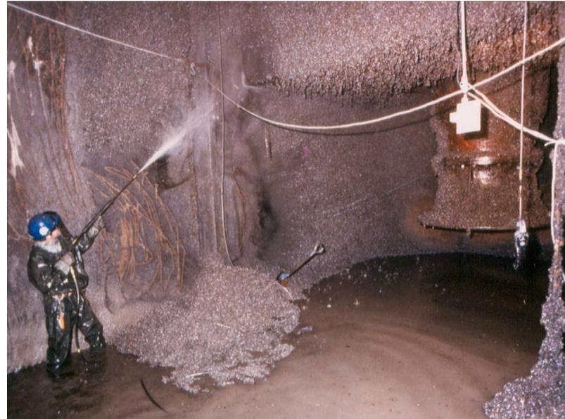
Zebra mussels, which arrived in the Great Lakes via ballast water discharge, clog power plant water intakes. Photo courtesy of DTE.
