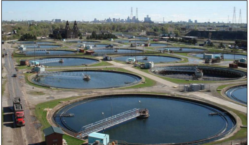
**Secondary or final clarifiers are critical assets at the Detroit WWTP. Detroit has 25 final clarifiers, with each clarifier 200 feet in diameter and a treatment capacity of 40.4 million gallons per day (MGD). The secondary clarifiers were constructed in stages from 1972 to 1979.**
