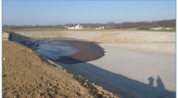
A recently constructed concrete lined manure storage structure at a dairy in Allegan County. This is one of two new structures the farm constructed to comply with the permit and make sure the structures are environmentally safe.
