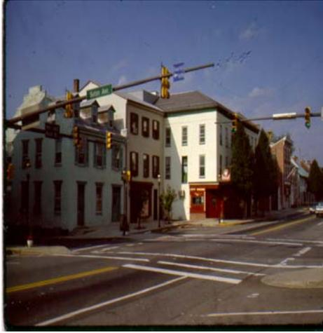
Other common terms applied to Type III or ordinary construction are "Main Street USA," and a "Taxpayer." The term "Taxpayer" evolved from "Main Street USA," where a building owner would operate a retail store on the first floor and live in an apartment on the second floor. It was said that the property taxes for the building were paid for by the store's income, and the shop owner lived above the store tax free.
