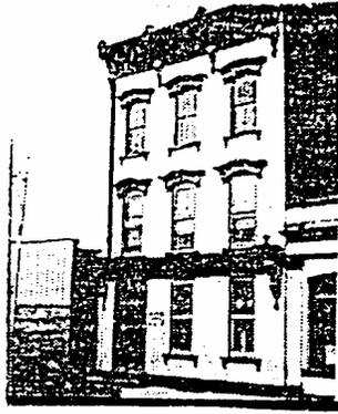
Buildings of ordinary construction generally are built no taller than six to eight stories due to the thickness of the supporting walls required to support the floor loads above the ground. The tallest building of ordinary construction is located in Chicago, Illinois, and is 15 stories high. Most ordinary-construction buildings on "Main Street" are only two or three stories high.
