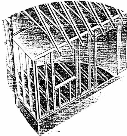
Another change in structural materials is the use of steel studs, which have become popular for many construction projects. Lightweight galvanized (to prevent rusting) sheet steel is formed easily into structural elements such as 2- by 4-inch or 2- by 6-inch wall studs. These noncombustible studs are stamped to provide openings for services such as electrical wiring and waterlines to pass through. One special risk is that the wall stud is an excellent conductor of
