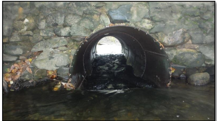
One of the improperly sized culverts on the North Branch of the Platte River, which limits fish passage and will be remediated.
