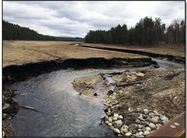
Incised channels in the former Song of the Morning Impoundment will be remediated.
