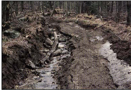
Figure 18. Forest Road Rutting Damage
