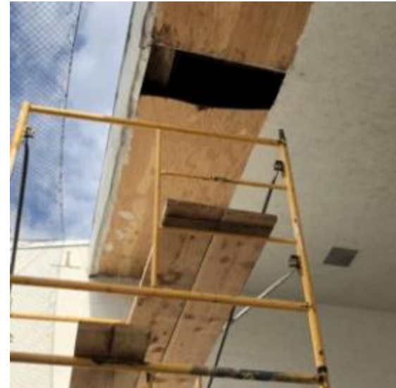
Handball Courts – deteriorated ceiling and roof trusses
