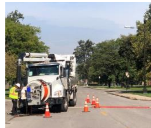
Combined Sewer System Inspection and cleaning
