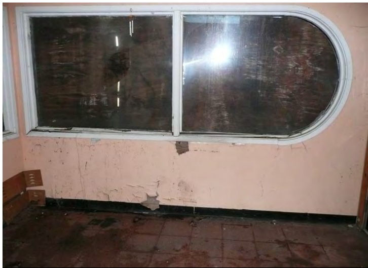
Damage Wall Board and Rotted Window Frames
