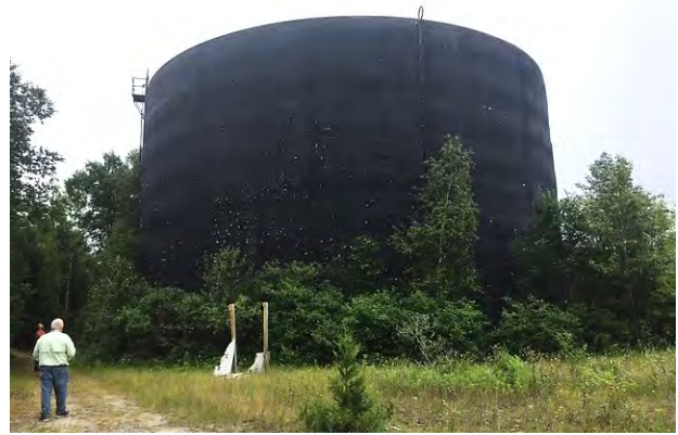
Two 1.75 million gallon fuel tanks dominate the landscape
