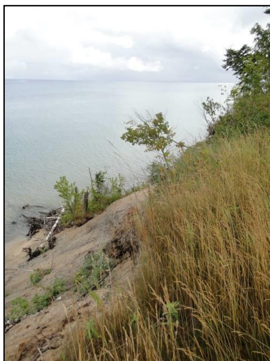
Erosion along the park's Lake Superior shore.
