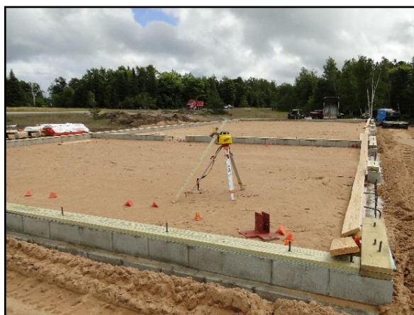
Construction of new park headquarters forced to relocate due to erosion, summer 2015.
