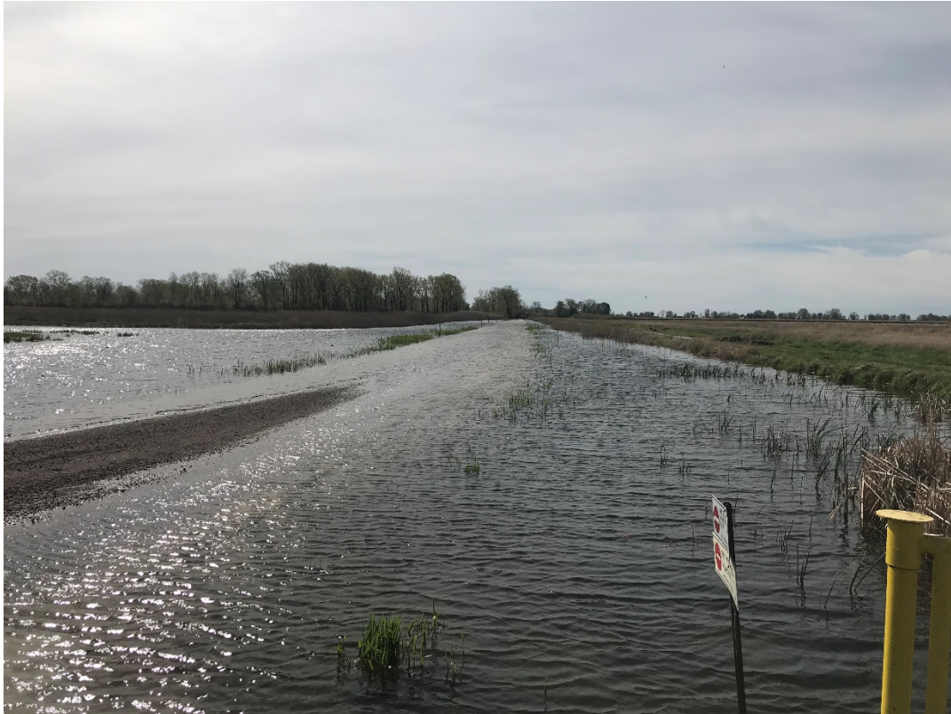
Voakes road flooded over, May 20. Photo by J. Darling
