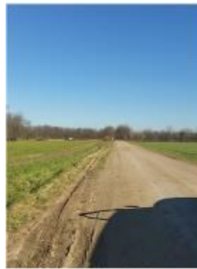
1800 ft of buried cable and new cable
