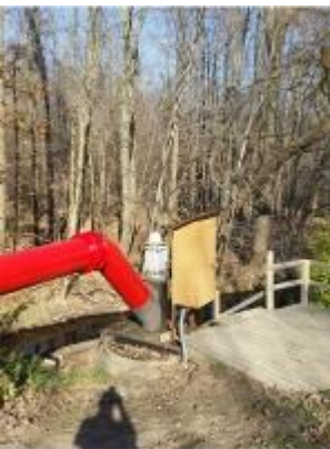
New base casting into hole
