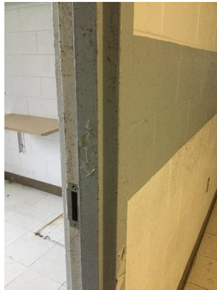
Description: Typical mold growth on cell door frames
