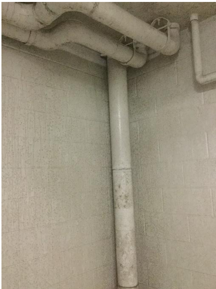
Description: Mold growth on walls
