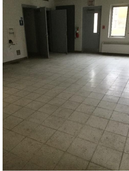
Description: Mold growth on visiting area floor
