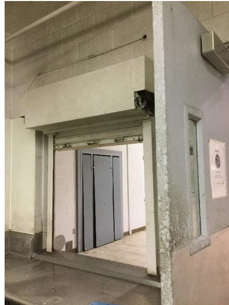
Description: Mold growth in kitchen
