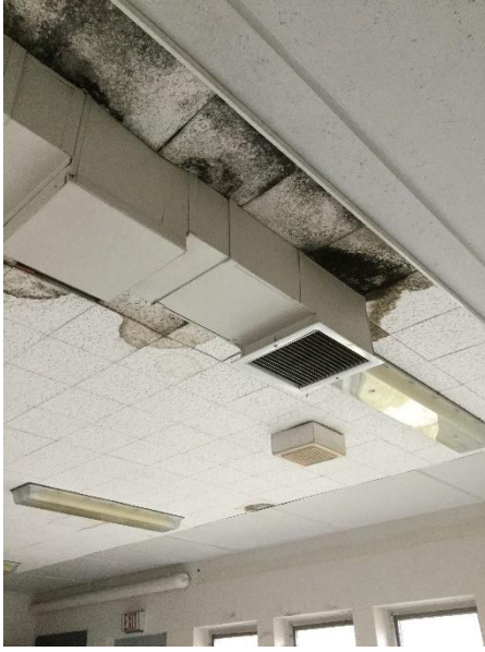
Description: Heavy mold growth and water damage in visiting area
