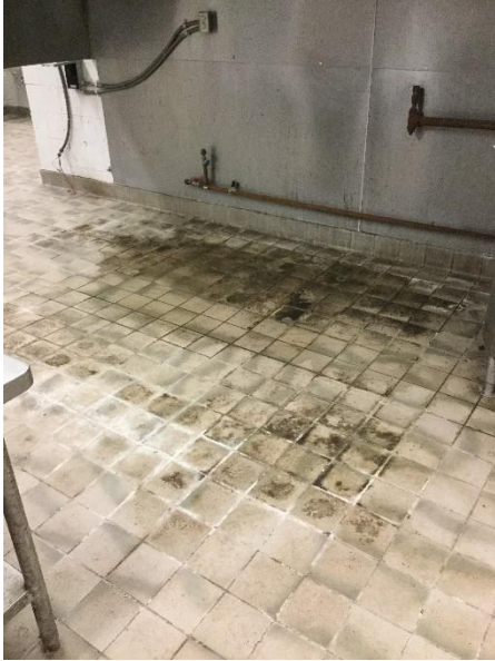
Description: Mold growth on kitchen floor Date: 10/9/2018 Taken By: AGK
