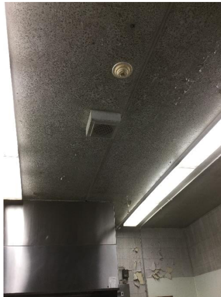
Description: Mold growth on kitchen ceiling
