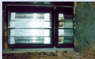
Photo 4C: Moldy air duct
