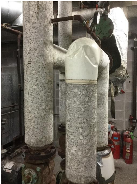
Description: Mold growth on mechanical room pipe insulation Date: 10/9/2018 Taken By: AGK
