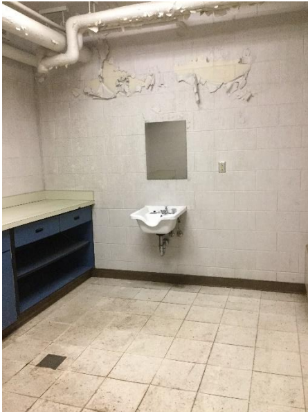
Description: Mold growth in barber shop
