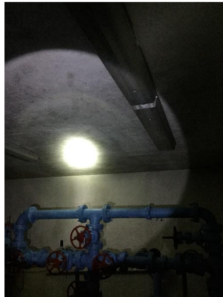
Description: Mold growth on ceiling of sewage treatment plant basement Date: 10/9/2018 Taken By: AGK
