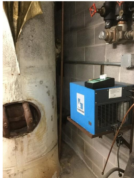
Description: Sample location in Mechanical Room Date: 10/9/2018 Taken By: AGK
