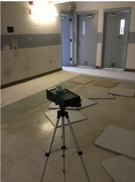
Description: Sample Location Cell Wing 2 Date: 10/9/2018 Taken By: AGK
