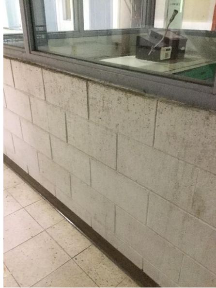
Description: Mold growth on exterior wall of security pod
