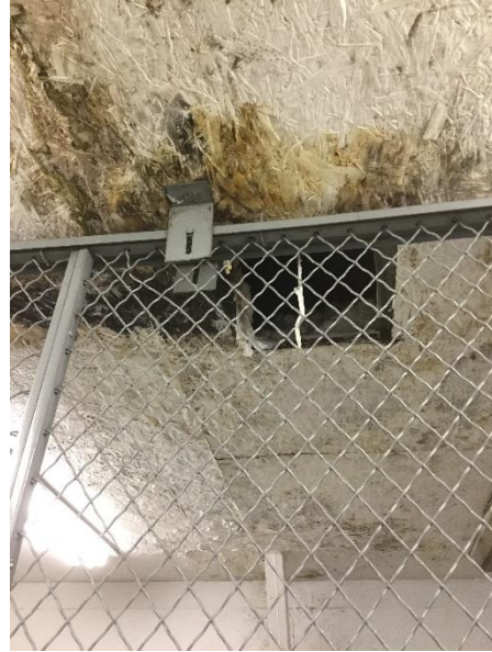
Description: Significant water intrusion in Maintenance Shop
