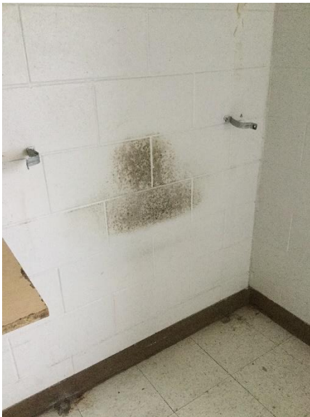
Description: Typical minimum mold growth in cells
