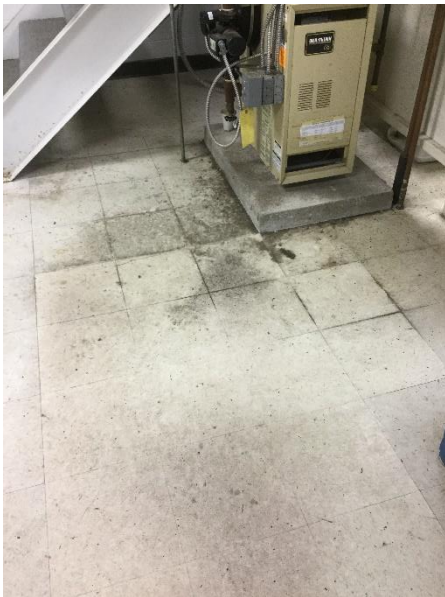
Description: Mold growth on floor of sewage treatment plant
