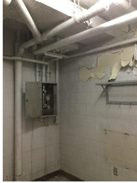
Description: Mold growth and indication of significant humidity damage in janitor closet
