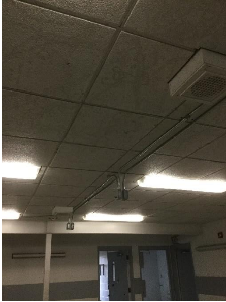
Description: Mold growth on ceiling tiles in cell wing common area
