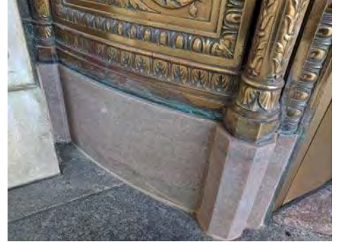
Picture 10: After Stone Repairs
