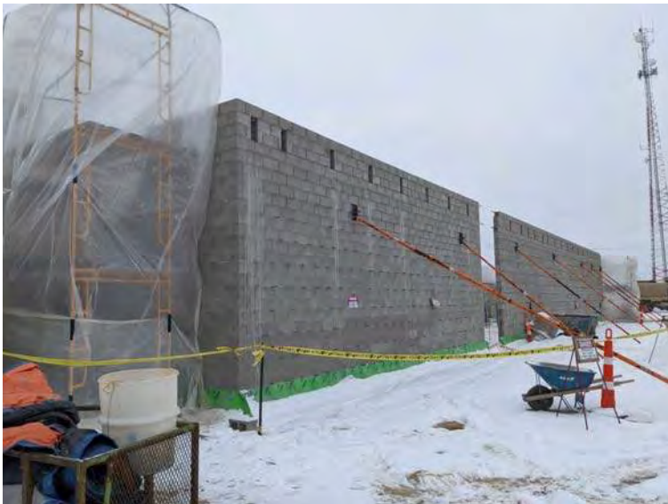
North Wall Addition
