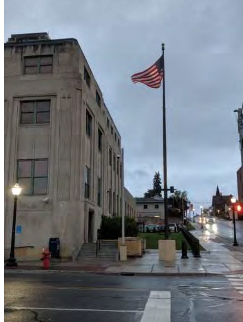
Photo 2: Bollards and Flagpole After
