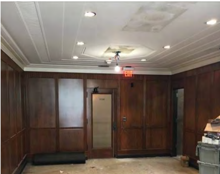
Photo 5: Walnut wall panels restored in the Library.
