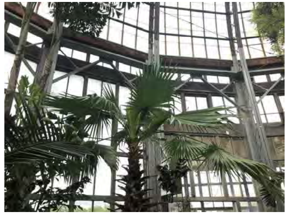
Picture 4: Conservatory Repaired
