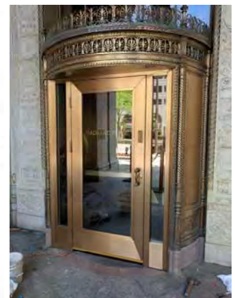
Picture 2: New exterior door rotunda
