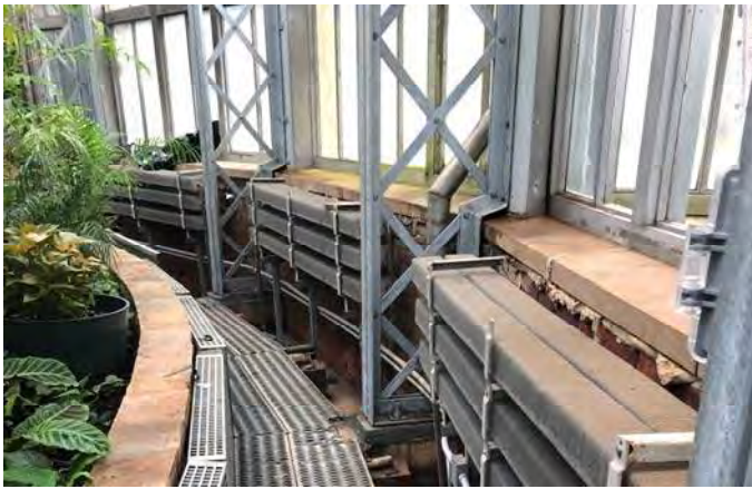
Picture 3: Column Base
