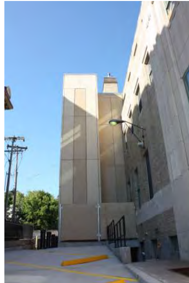
Photo 2: Elevator Tower Addition.
