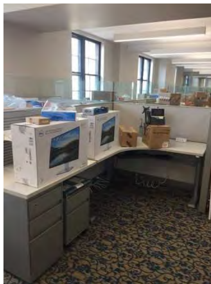
Restored ceiling height
