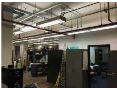
Pre-Demolition O&M Space
