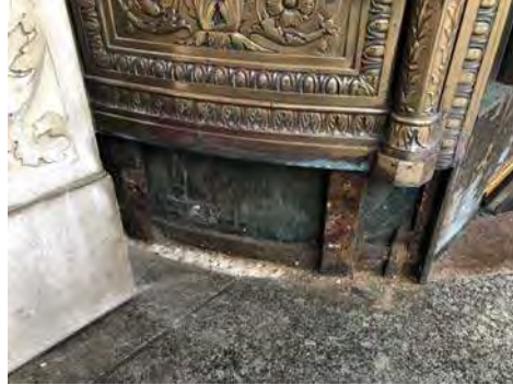
Picture 9: During Stone Repairs
