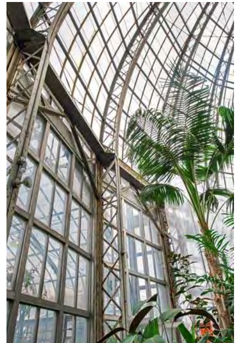
Picture 2: Original truss column in the Palm House
