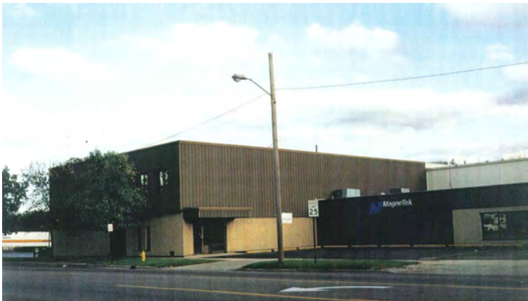
Above - MagneTek Facility prior to demolition.
