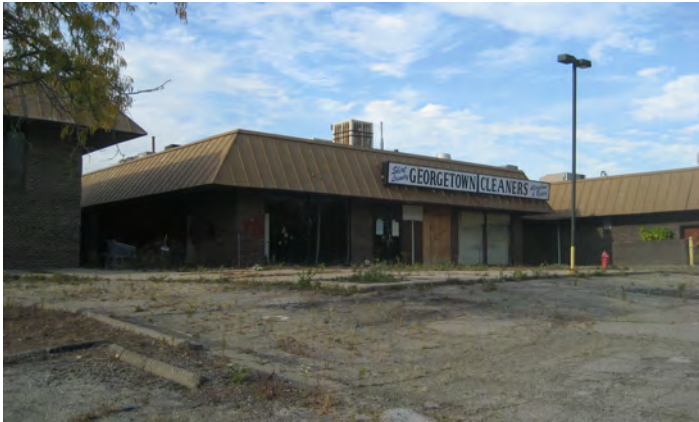
Above - View of Georgetown Cleaners pre-demolition.
