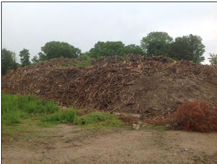
Stockpiled debris - Former Whitehall Leather Company - Whitehall, Michigan (2018)
