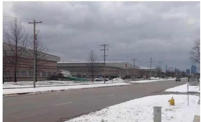
Above - 2018 view of warehouse buildings.
