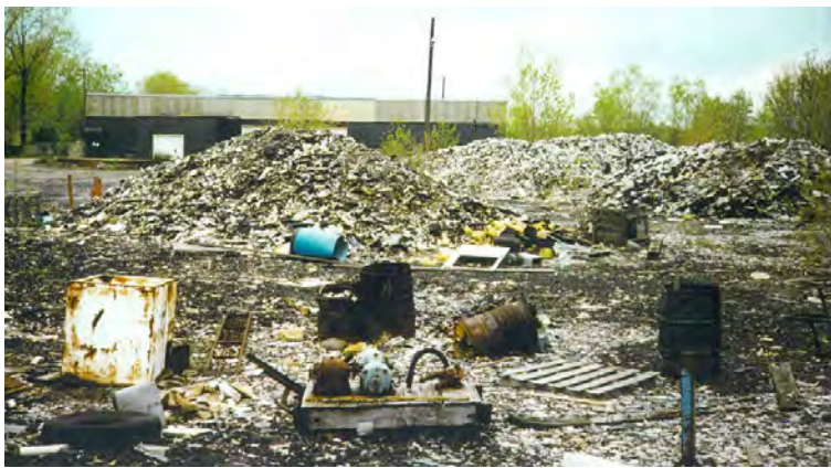
Above - View prior to cleanup activities.
