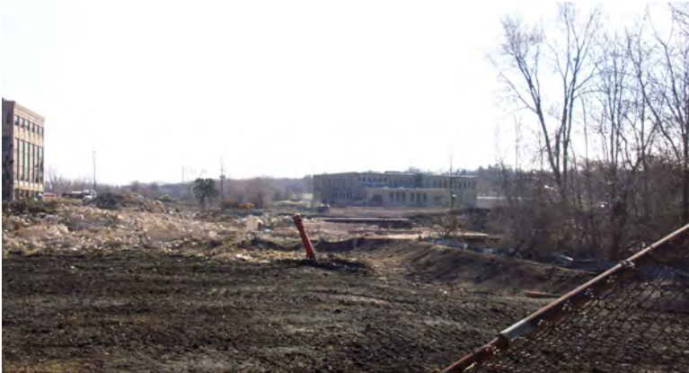
Above - 2005 View of Performance Paper Demolition.
