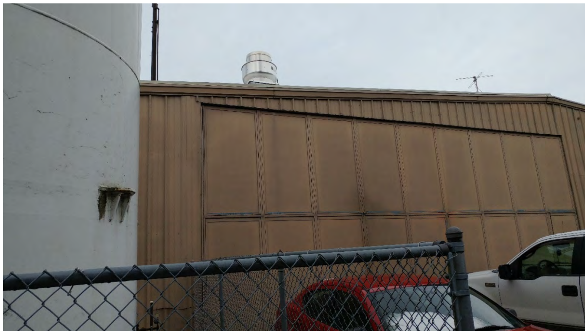
Figure 7 – Containment Room Vent
