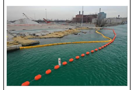
Cable buoys, erosion control blankets, and 5-foot turbidity curtains – facing north/northwest.
